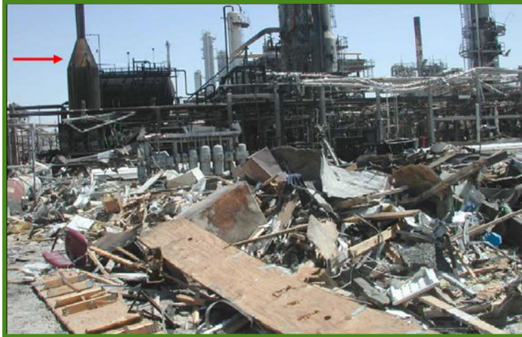
BP Texas City Explosion
